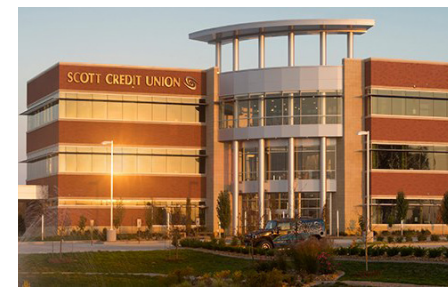
HOME OFFICE 101 Credit Union Way in Edwardsville, IL October, 2012; LEED Certified Building
